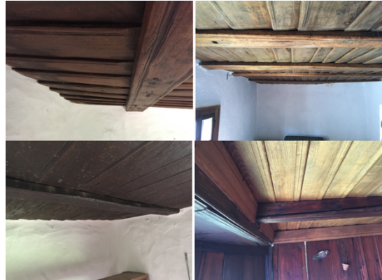
Figure 12: Wooden ceilings („šiše“) on the premises
