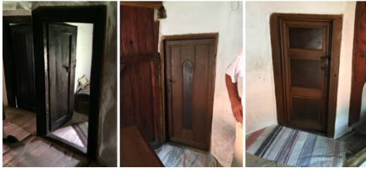
Figure 15: Doors in rooms next to the open fireplace (left) and doors in chardaks (center and right)
