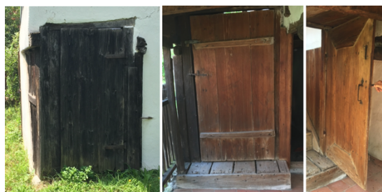
Figure 14: Doors on access stairways for first floor
