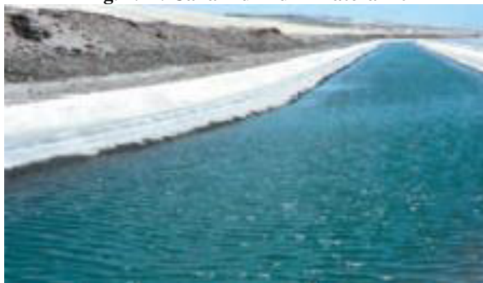
Fig. 2.12: Canal Pur Pur – Lateral 10
