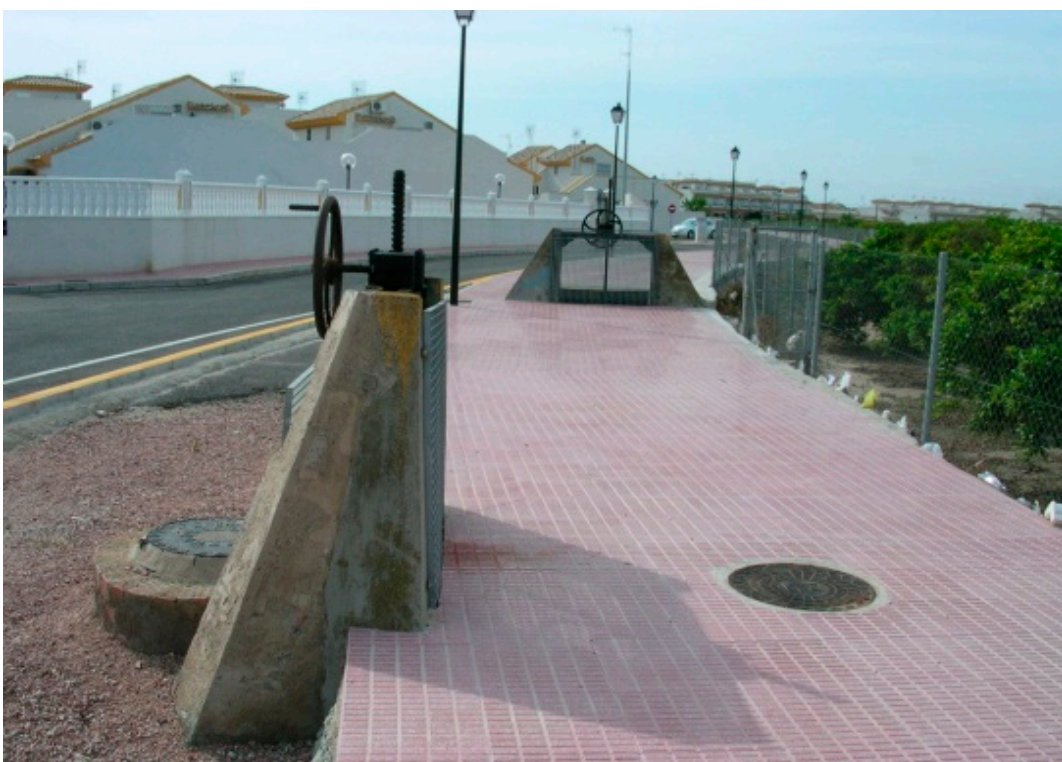
Figure 4. Main canal in Formentera village. The advance of residential use has motivated the concealment of the hydraulic infrastructure under the ground, essential for the survival of the Orchard. Author: Gregorio Canales-Martínez.
