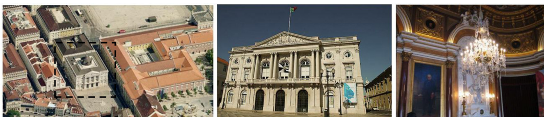
Fig. 3. The historical building (Lisbon City Hall).
