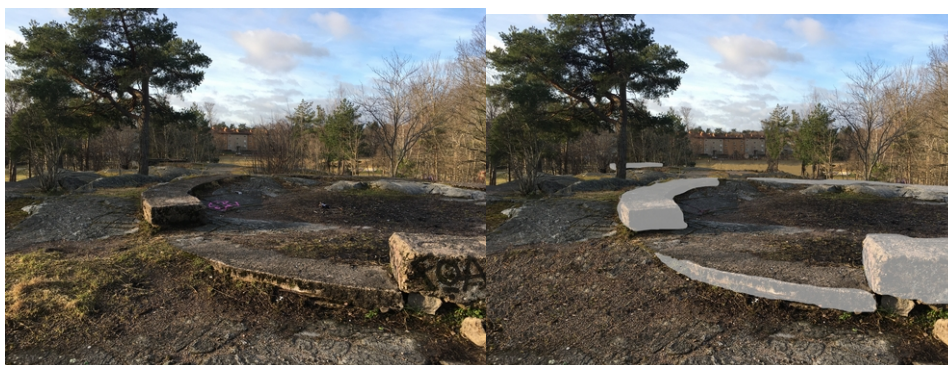
Figure 5 (left, as now). Figure 6 (right, proposed): Views have been opened up, rubbish removed, paint applied. Photograph: Richold, J (2020)
