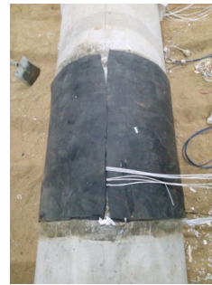
Fig. 5. Sponge rubber around the tunnel
