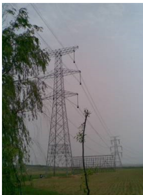
Fig. 4. SZ21-type tangent transmission tower in Liaoning province, China
