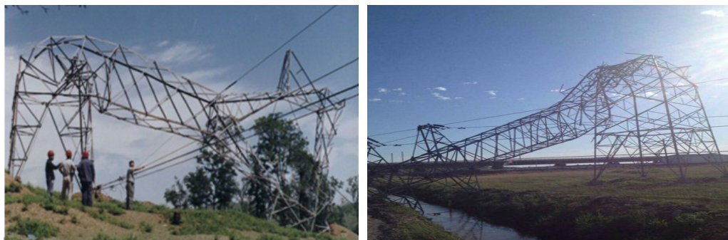
Fig. 1. Wind induced collapse of transmission towers
