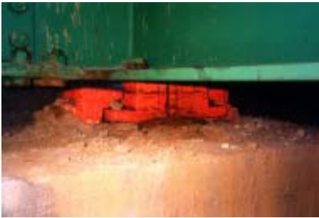
Fig. 1. Spherical bearing (Park, Chang-Ho, 2008)
