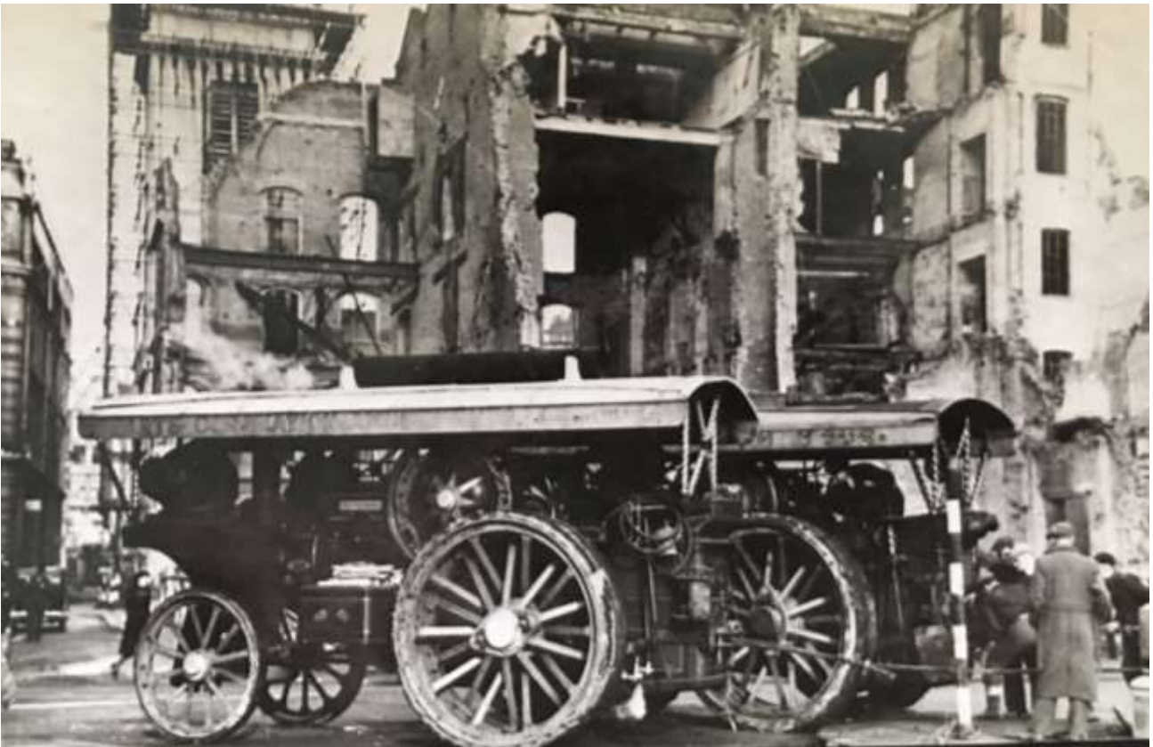
Appendix M – Fowler 8NHP Showman’s Engine ‘The Princess’ No. 14868 built in 1917 in the foreground with what is believed to be Fowler No. 14902 in the background. Both engines on demolition work in London, likely in 1942 when Philip Bradley records seeing 14902 at work. Photograph from authors collection.
