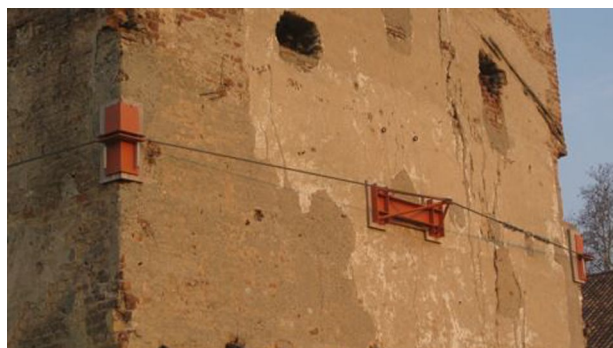
Fig. 1 An example of a provisional intervention aimed at preventing the out-of-plane rocking of the façade
