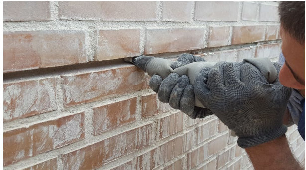
Fig. 9 A mastic gun was used before and after the application of the steel cable for joint repointing
