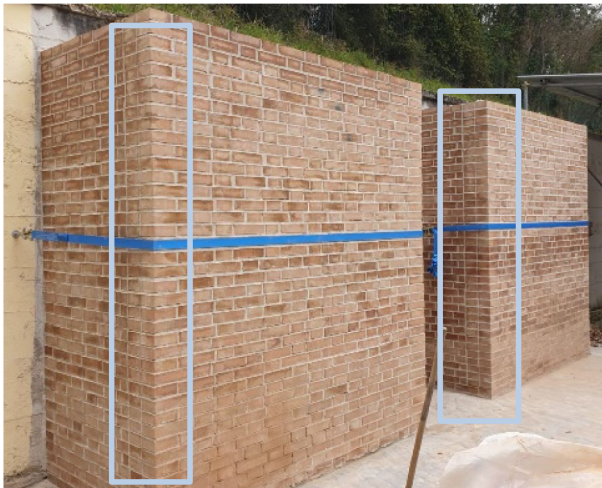
Fig. 4 The two C-shaped brickwork specimens. In the two boxes, it can be noted the vertical mortar joint used to connect the wall panels at the edges [the blue strip was only used during curing time for safety constraints]
