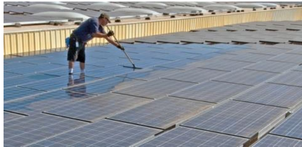
Fig. 1.19- Cleaning the soiling in a PV array
