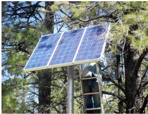
Fig. 1.21- Partial shading
