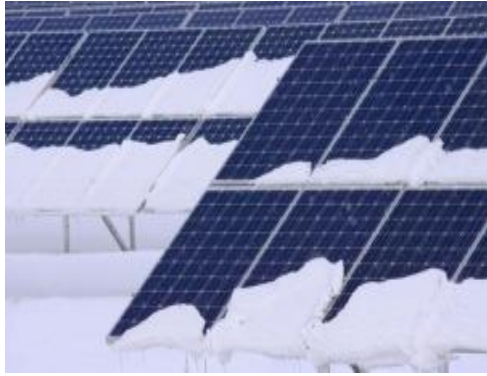
Fig. 1.20- Snow covering PV modules
