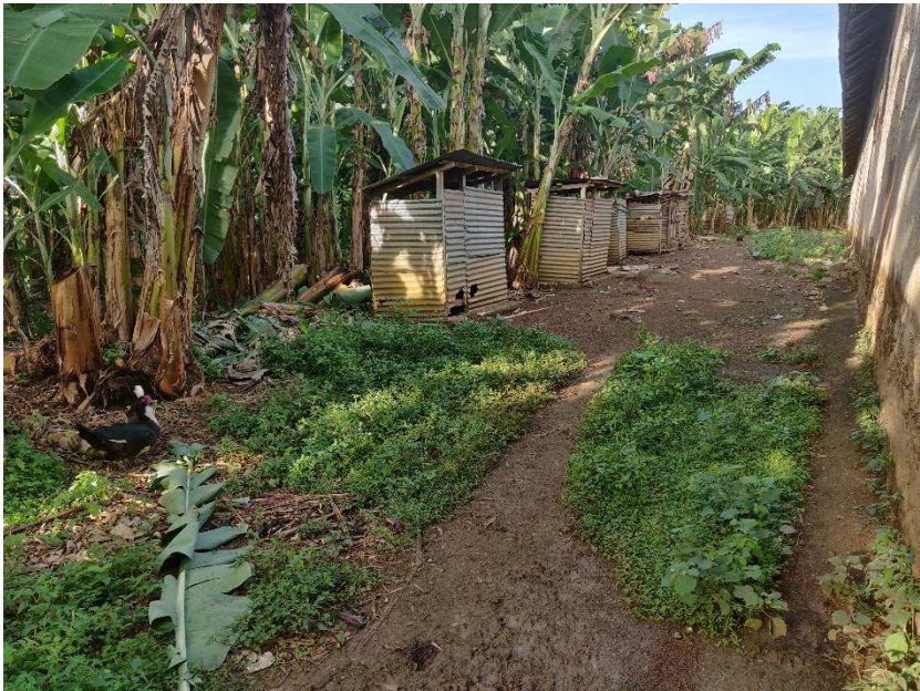
Figure 6: three latrines in Plancas in disrepair and unused.
