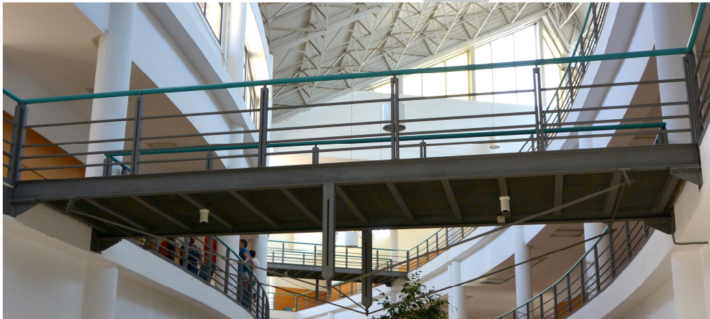
Figure 6. General view of the pedestrian bridge used for the experiment. A person jumping in the center excites the structure. An accelerometer in the upper part of the deck will register the main vibration.
