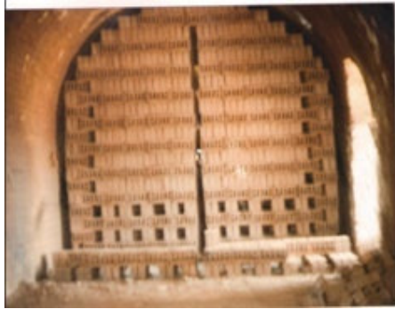
Plate 4 Fired red bricks before using the suction pipes (Faint Red Color)
