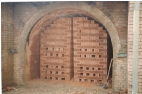
Plate 5 Fired red bricks after using the suction pipes (well fired with red color)
