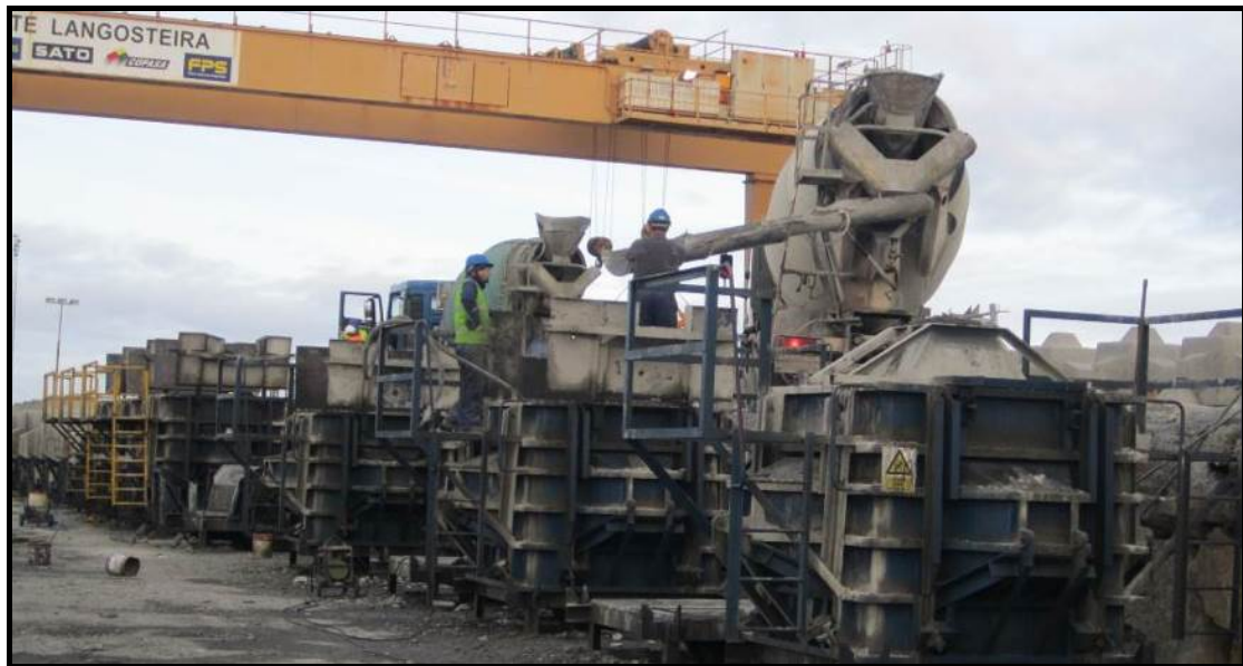
Figure 7. Production line of 25-tonne Cubipod units.
