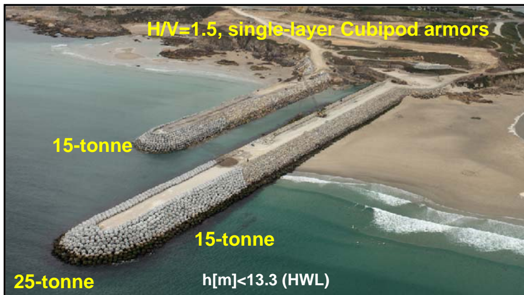
Figure 10. Single-layer 25- and 15-tonne armors in the southern breakwater and the northern groin at the end of July 2013 at Punta Langosteira (A Coruña, Spain).
