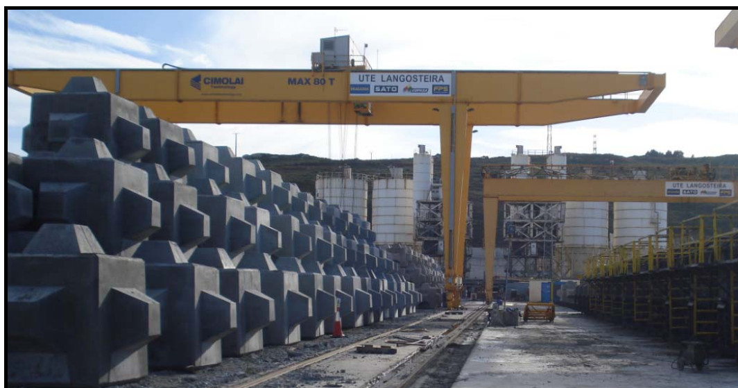
Figure 6. Block yard, gantry cranes and stacking of 15-tonne and 25-tonne Cubipod units in three levels.
