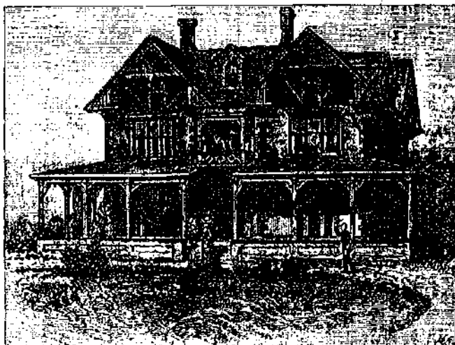
ADOBE RESIDENCE AT RIVERSIDE.
