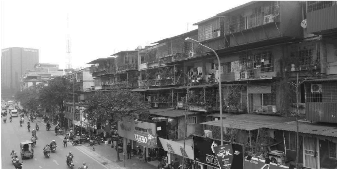
Figure 1. Block of flats with extensions in Hanoi city, Vietnam
