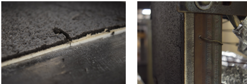
Figure 10. Details of the final intumescent char (sample CP-HSC3-01).
