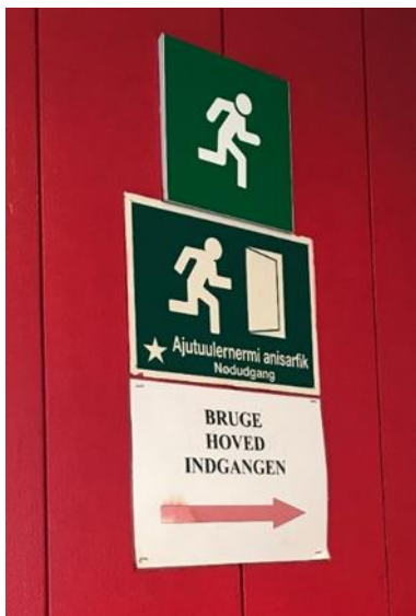
Figure 22. Emergency exit sign at Nuuk airport
