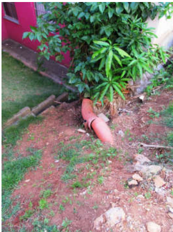
8-7 Pipe mentioned when discussing potential issues around the area
