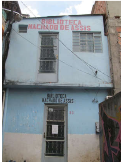
8-15 Door on the upper floor at the local library Source: picture taken by a respondent, 2016.
