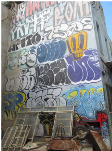
8-25 Side wall - Community Centre
