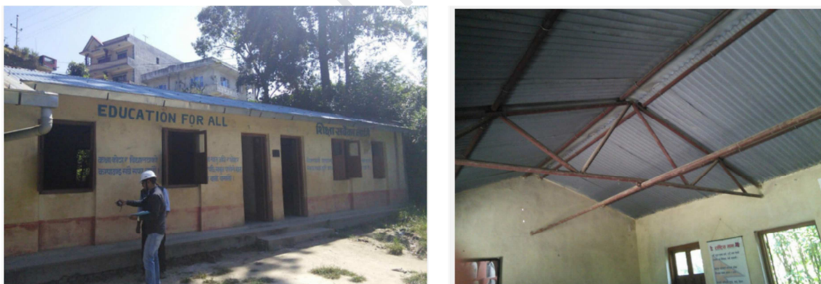
416 417 Figure 5. Photographs representative of an IB of the UCM-URM7/LR(1)/LD school building type: (left) outside 418 front view and (right) Inside view showing the flexible roof diaphragm. (Photo from Nepal, Copyright: The 419 World Bank).
