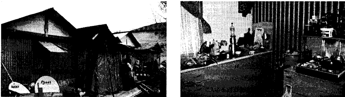
Figure 39 Two paper temporary houses are consolidated into one dwelling with the addition of a kitchen and bathroom in the middle. Outside view of the house (left) and inside view of the kitchen built between the two paper houses (right).
