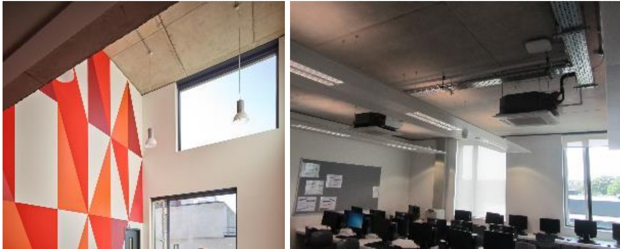
Figure 10 Exposed concrete ceiling in common areas and classrooms
