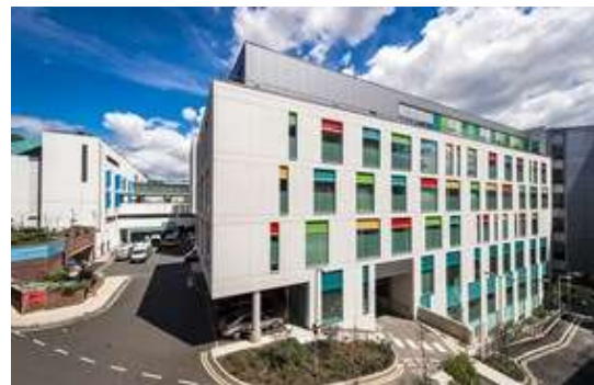
Figure 1: Case study hospital building
