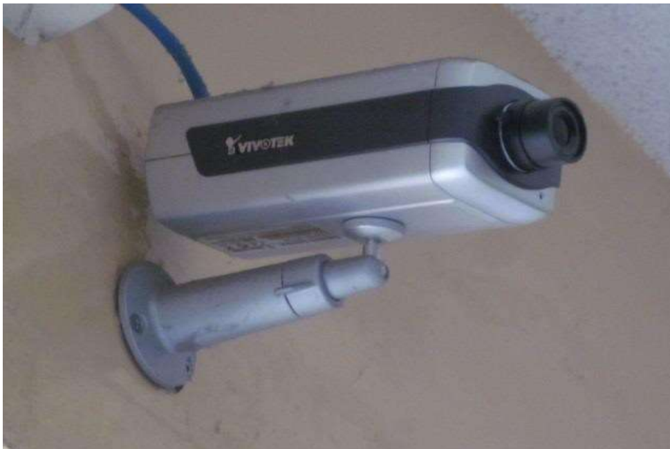
CCTV surveillance still in operation: both safety and discipline
