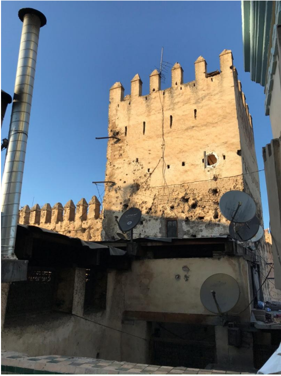
Fig. 6: Details of the earthen masonry of a fortified structure (northern district).
