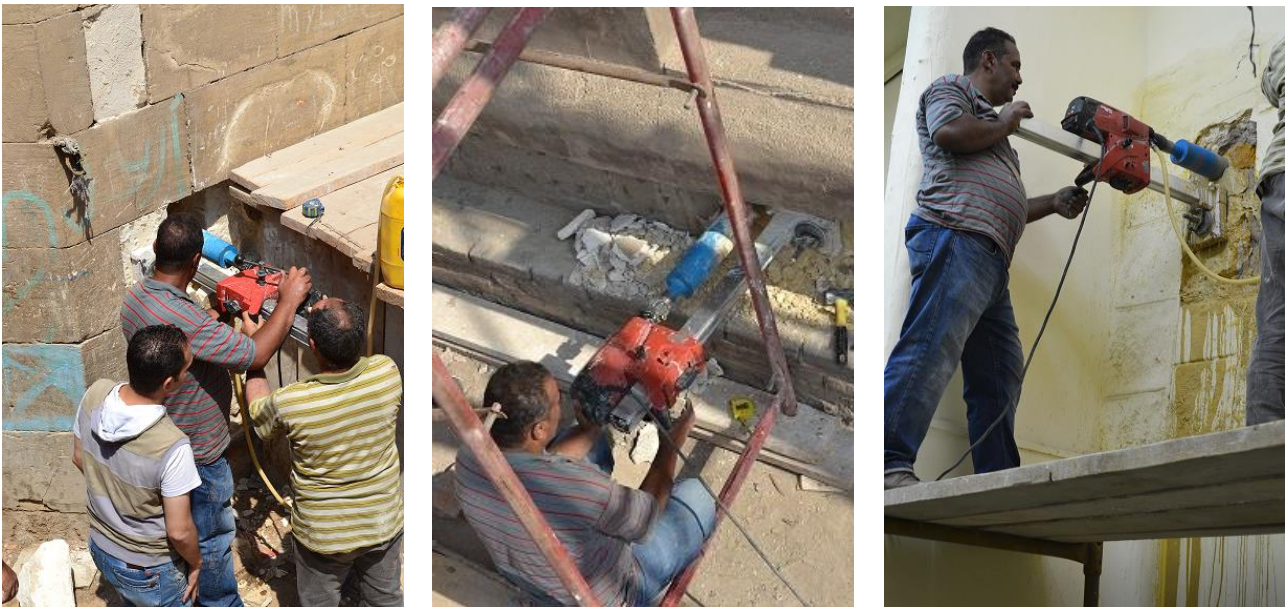
Figure 5. Extracting of the investigated core samples
