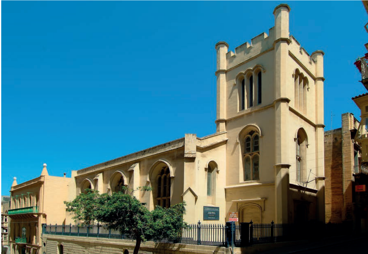
St Andrew's Presbyterian church in South Street, built in a Neo-Gothic style by architect Giuseppe Bonavia in the late 1850s
