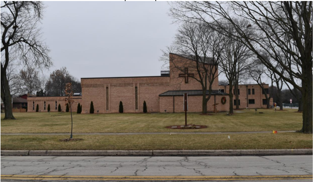
Figure 3-2: St. Thomas Becket as viewed from the street. During most of the year, leaves would further block the view of the church from the street.
