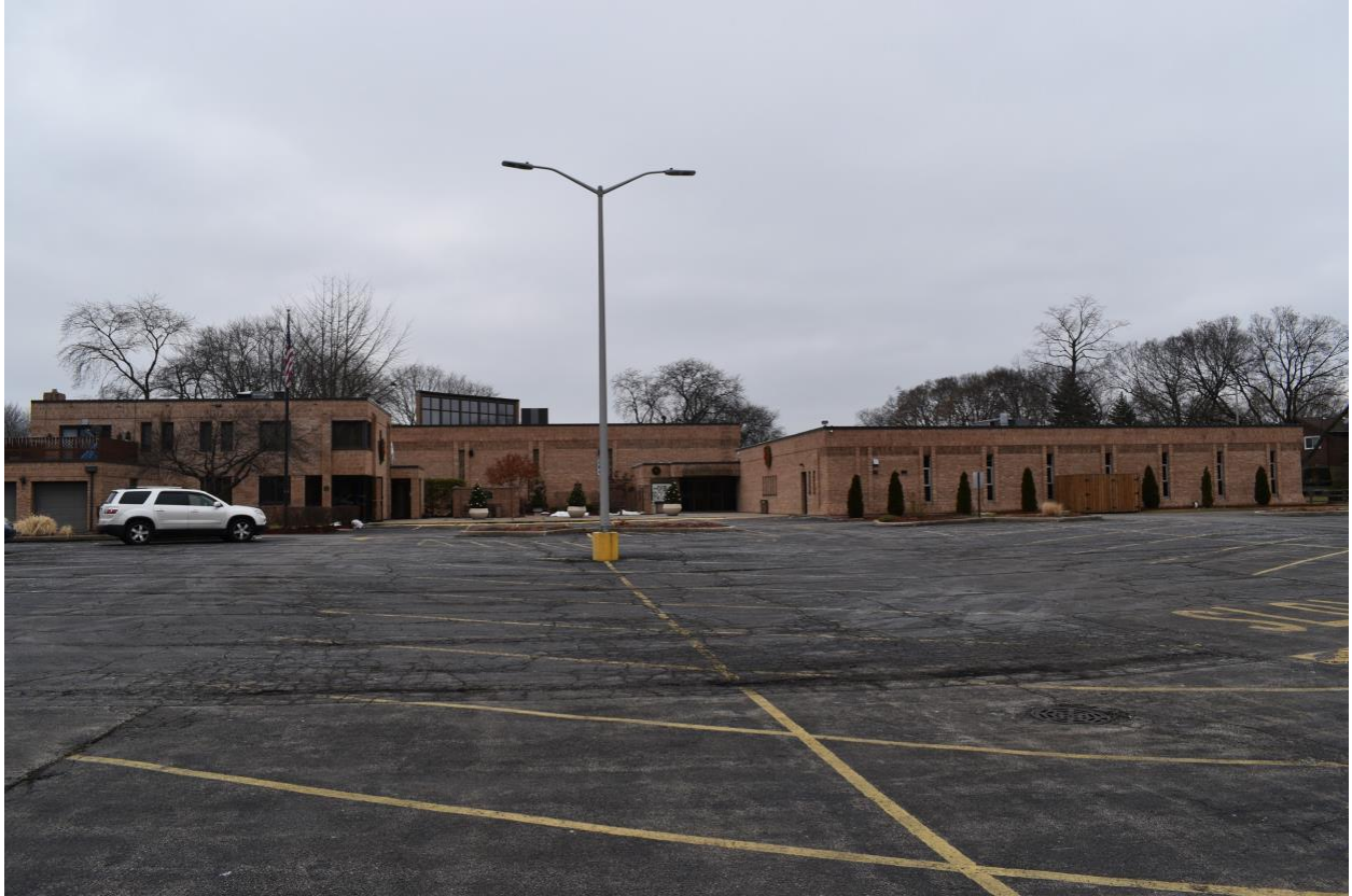
Figure 3-3: St. Thomas Becket as seen from the parking lot.
