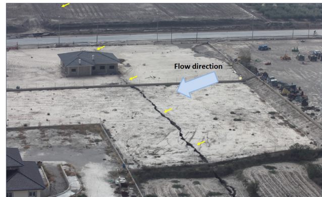
Figure 4. Aerial view of the northern section of the crack (courtesy of Puerto Lumbreras City Council). The yellow arrows indicate the location of the earth fissure (modified from Mulas, 2013).
