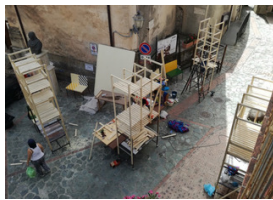
<INSERT Fig. 13: Construction during summer workshop 2018>
