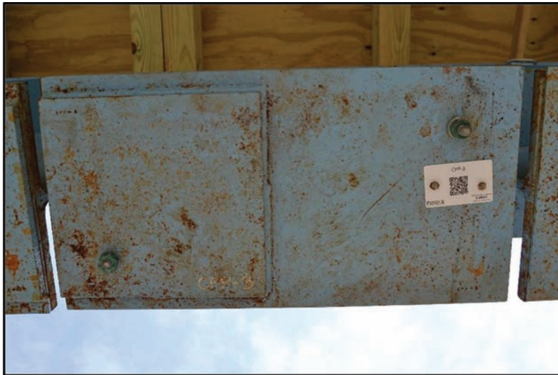
Figure 6 Welded cover plate specimen.
