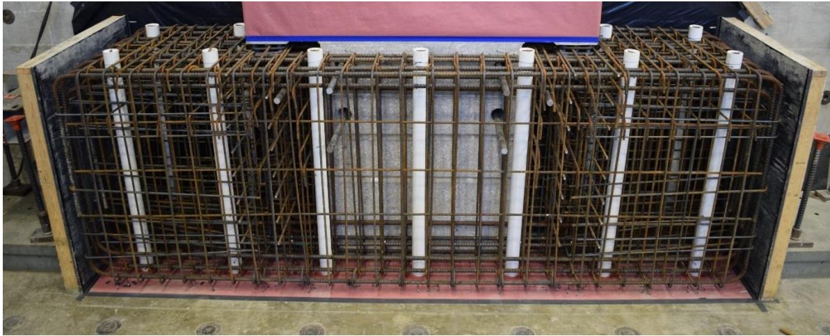
Figure 28 – Reinforcement in Wall Foundation – Side View.
