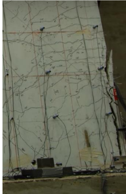
Figure 10 –Splitting cracks in lap splice in Specimen PW1 by Birely (2012).
