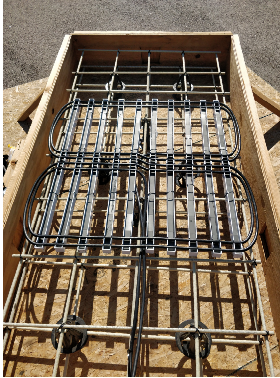
Fig. 3.1: Induction coils before concrete was poured
