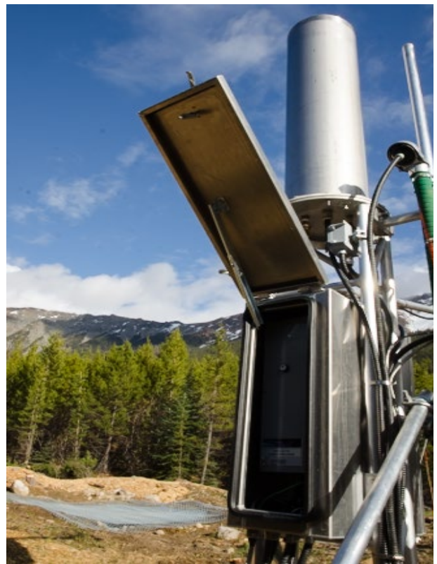
Figure 3.14 Custom-built snow pillow with open hydraulic system and submersible pressure transducer.
