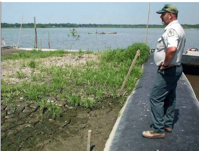
Figure 13. A DNR site manager stands on a geotube in August. The sediment is well consolidated and supports volunteer vegetation. Plants began growing on the island after the first week, but were generally eaten by waterfowl or killed by high water. The geotubes successfully protected the island from erosion during the summer and fall, despite frequent water level fluctuations and high winds.
