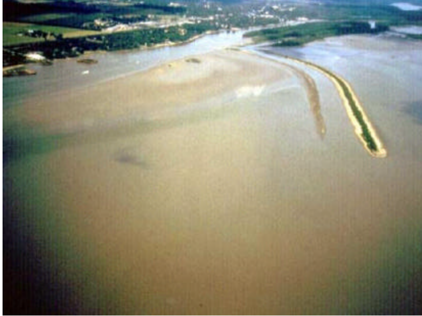
Figure 5. Island in Upper Peoria Lake four years after being constructed with a clam shell bucket. The island to the east (right) is about six feet high and supports vegetation. It was built with deeper sediment and contains some sand from the original bottom. The west island is composed totally of soft sediment and was originally about two feet high. The navigation channel is at the top of the picture. This part of the lake is about 1.5 miles wide and about approximately a foot deep.
