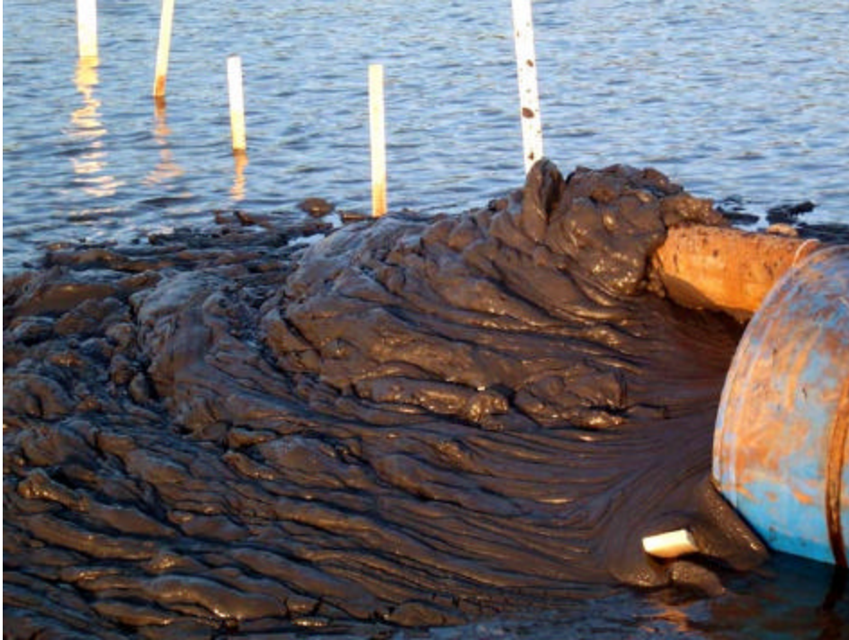
Figure 7. Sediment discharged by the DRY DREdge™ in upper Peoria Lake maintained its original moisture content and readily formed piles with about a 1:9 slope. The dredge used a positive displacement pump to move clam shelled material.
