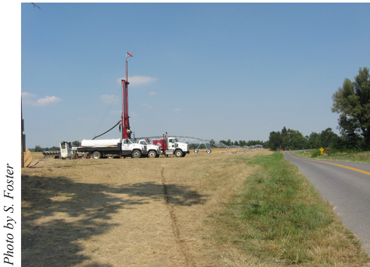
Figure 5a. Irrigation system being installed June 25, 2012 in aquifer of unconsolidated sediments in Carlisle County.
