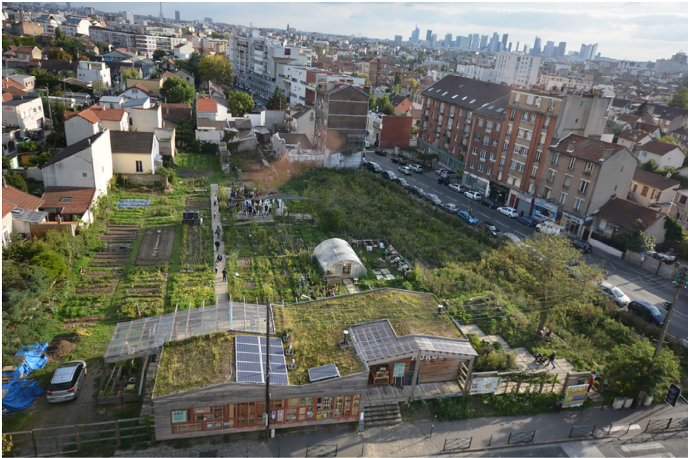
FIGURE 2 R-Urban AgroCité, Colombes Source: aaa [Color figure can be viewed at wileyonlinelibrary.com]
