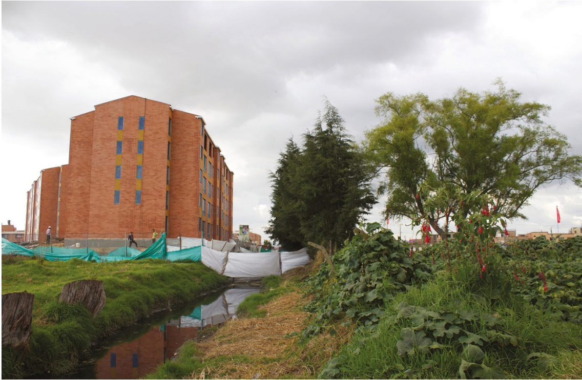
Figure 6. Low-cost housing project built along an agricultural canal.
