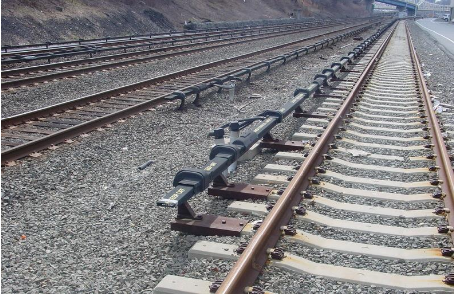
Figure 2. Third rail electrification system [8].
