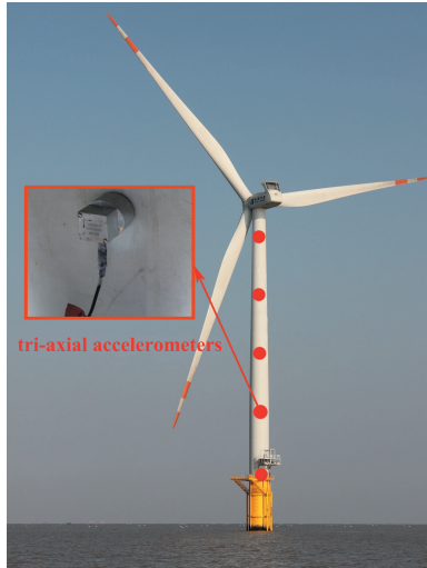
Fig. 19: Test offshore wind turbine.
