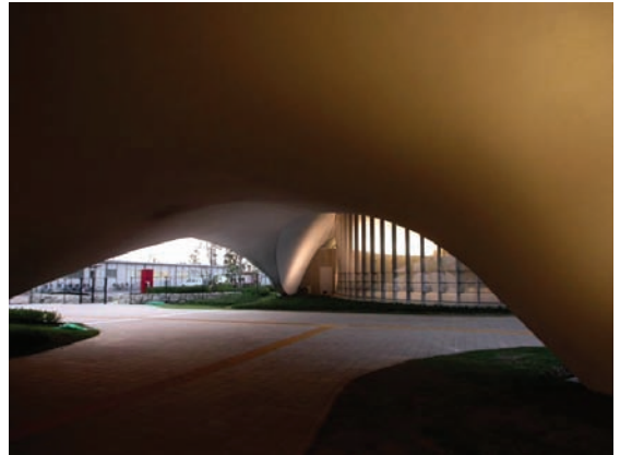
Figure 11: Fukuoka central “Grin Grin Park” roof by Toyo Ito 2005
