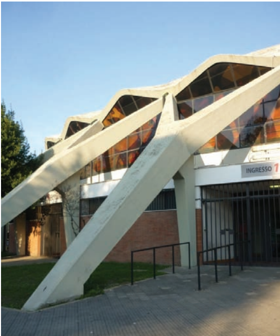
Figure 7: Y-shaped columns on the outside of Palazzetto dello Sport, Rome, Italy by PL Nervi (1956-1957)
