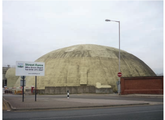
Figure 8: A grit salt storage made using pneumatic formwork, Sheffield UK
