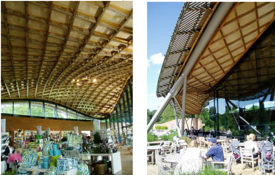
Figure 1a and b: The gridshell roof at The Savills Garden Gridshell
