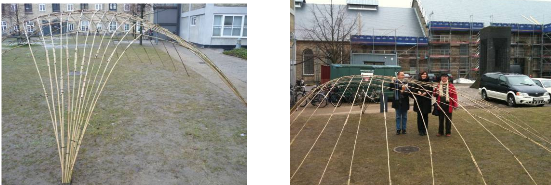
Figure 7a and b: The completed gridshell
