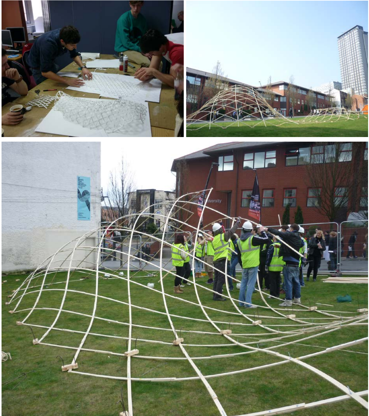
Figure 3: Physical models of timber gridshells were made from paper card strips (top left). The Swell timber gridshell (top right) on display for 2 weeks in Sheffield City Centre in 2011. Students create the shells together to learn and understand timber as a material in bending and deformational behavior arising from forces applied. (Bottom) [credit: Gabriel Tang]
