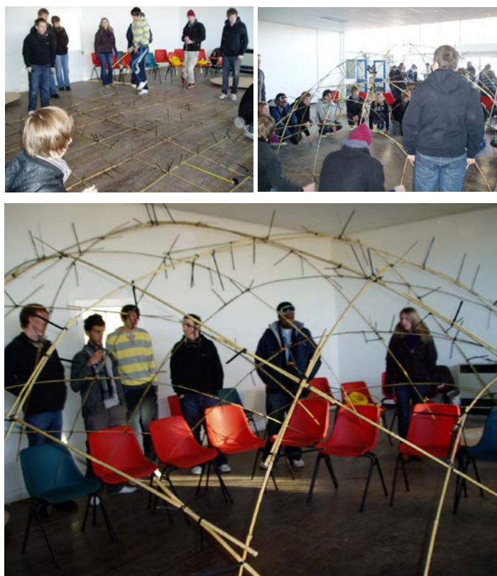
Figure 2: Bamboo gridshell construction workshop held in 2008 demonstrates the deformation of a flat mat to result in a anticlastic dome. [credit: Gabriel Tang]
