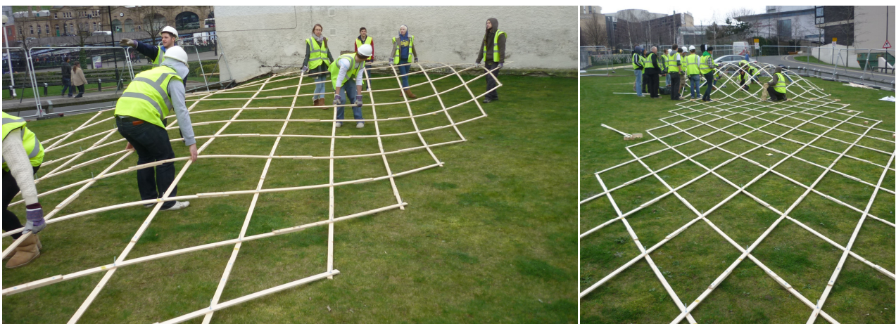
Fig6 a) Flat mat is carefully lifted and moved to correct orientation. b) the baby swell is visible at far end.
