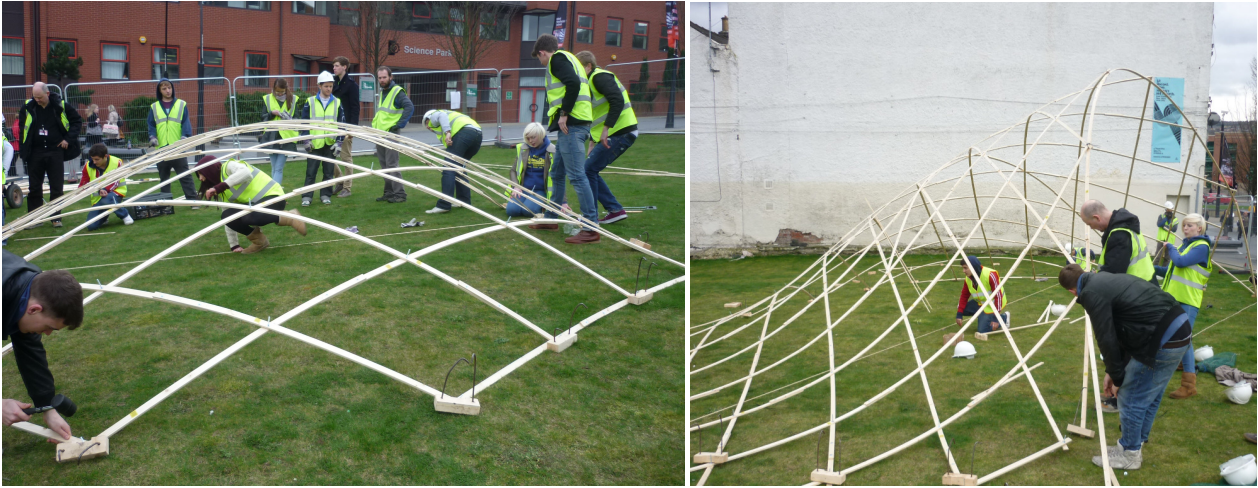
Fig 7. a) The baby swell is fixed by pegging down. B) Bracing members are fixed to triangulate grids to lock in form.
