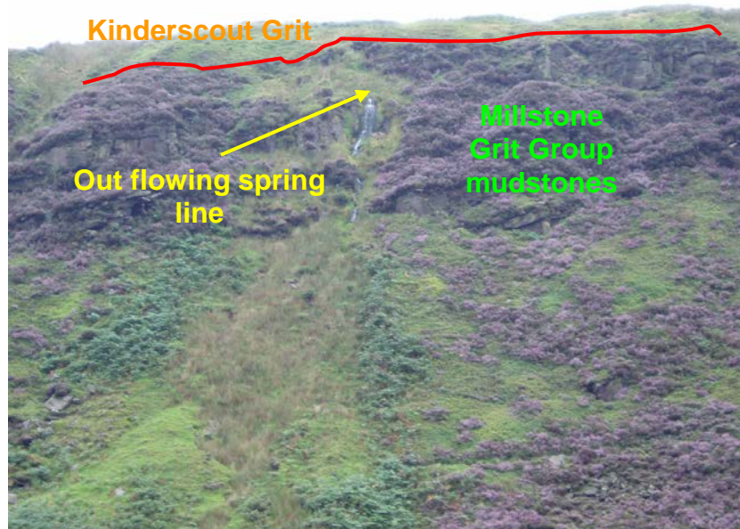
Figure 2.12 - A spring line out flowing just below the Kinderscout Grit and mudstone boundary on the rear scar of Rake's Rocks landslide (BNG 406198 400480 facing 230°).
