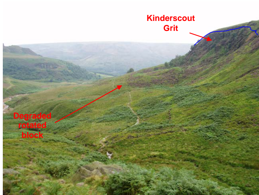
Figure 4.7 - View looking over to Black Tor Landslide (BNG 406180 400494 facing 150°)
