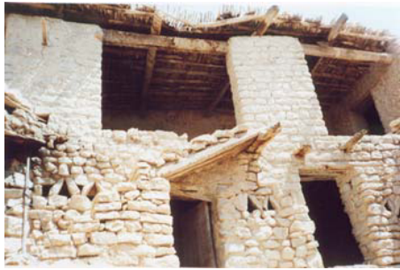
Figure 5: Whilst the upper floor spaces are widely opened to courtyard, the rooms at the ground floor are daylit by means of the door and small windows.
