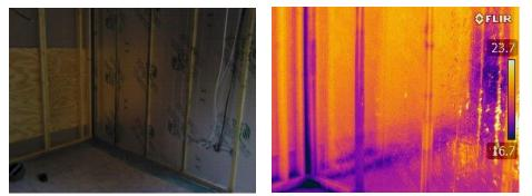
1st floor apartment – Internal view of external wall, West Façade. Ceiling to wall junction and window detail. (Bedroom) Digital Image 2 Junction detail Thermogram 2 Junction detail
