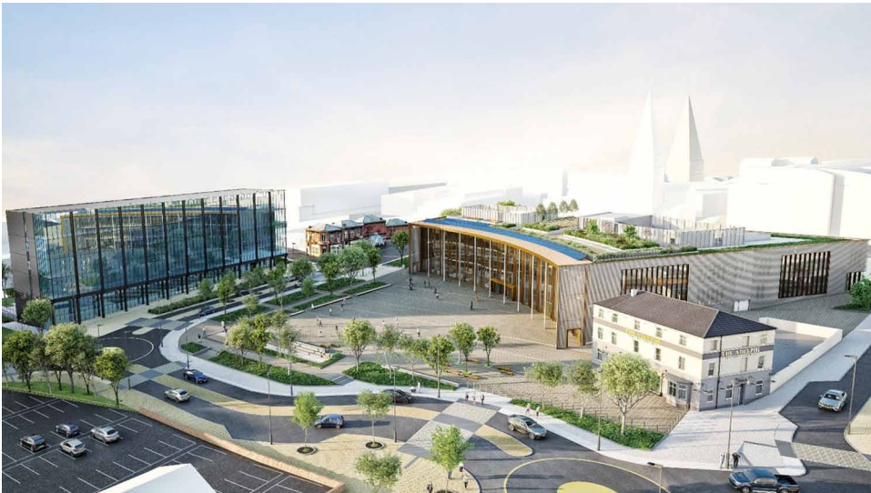
Figure 3. Image of the completed UCLan Masterplan Central Projects – Engineering Innovation Centre, Student Centre, Adelphi Square, & Highways Project
