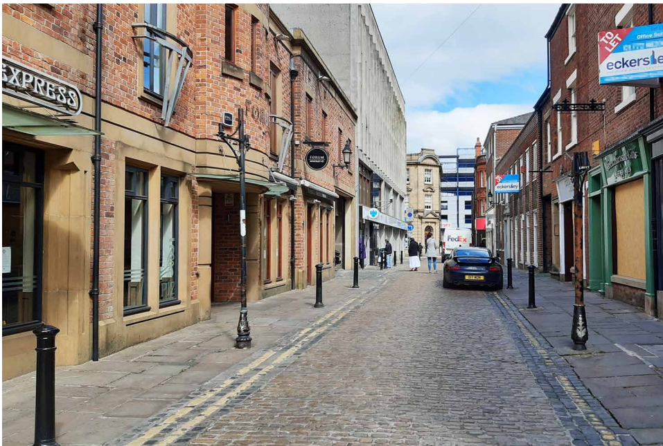
Figure 8. Image of Winckley Street, Preston illustrating level surface between footway and carriageway (©E. Kamel).
