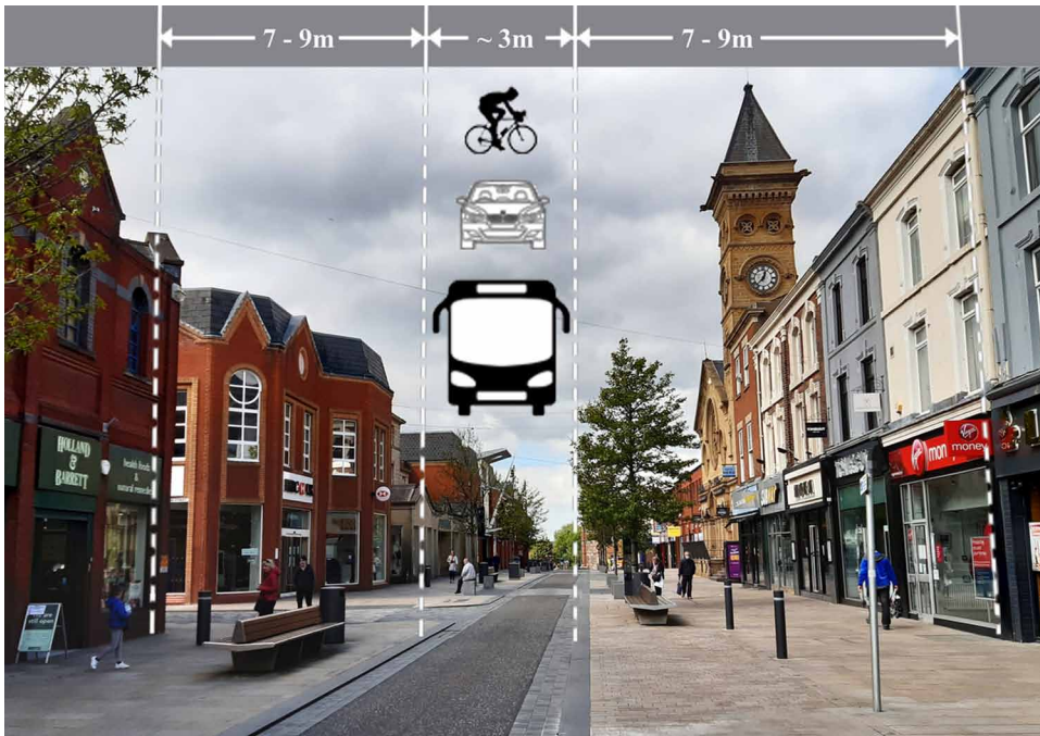
Figure 2. The completed Fishergate Central Gateway Project, including 'courtesy crossings' (©E. Kamel)
